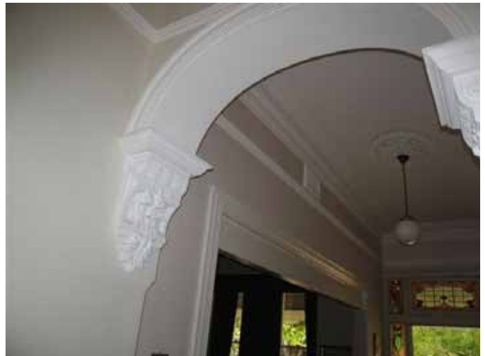
Ceiling detail of hallway
